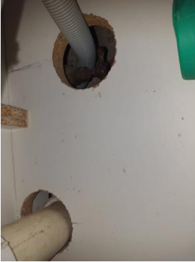
Mains Isolation Valve
