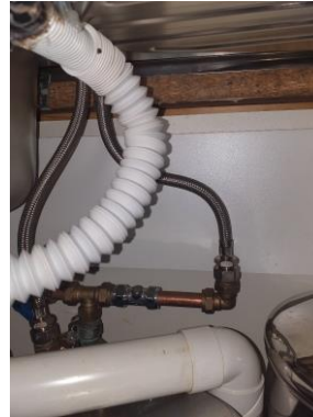
Representation of Flexible Hoses
